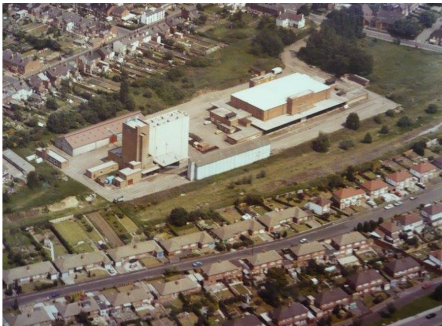
Aerial photograph of the cold storage unit in 1982 showing the site of the lifted railway sidings on the Bewdley Road side.
